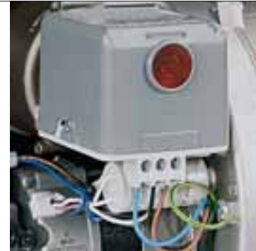
Control box fitted with an ignition transformer
